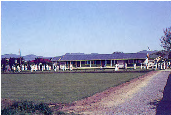
The new Bowling Club pavilion completed . . . 19 weeks later.
