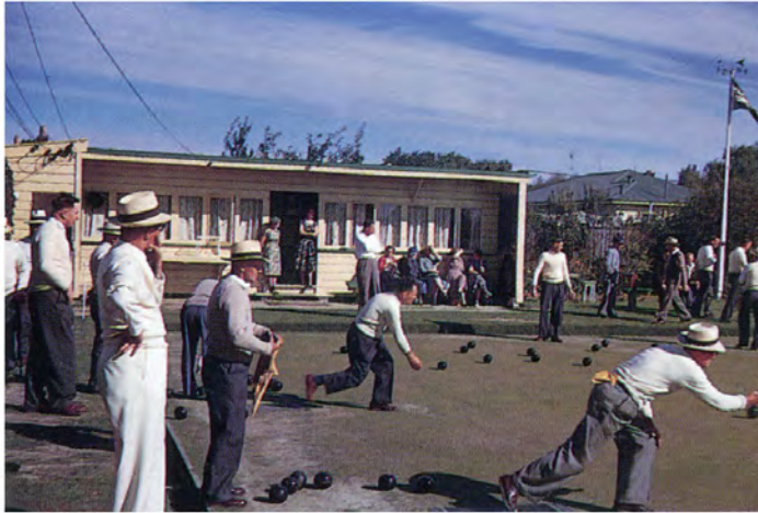
The original Bowling Club pavilion.
